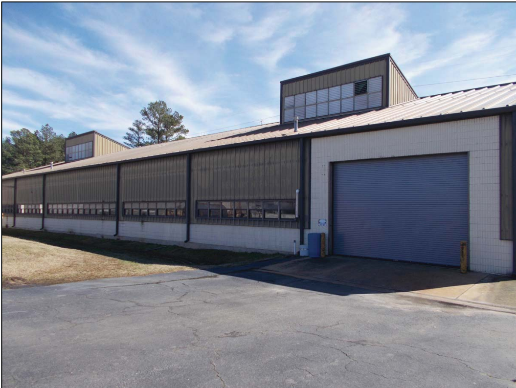
Figure 5-29. Building 62, north façade, view southeast (DSCN1583).
