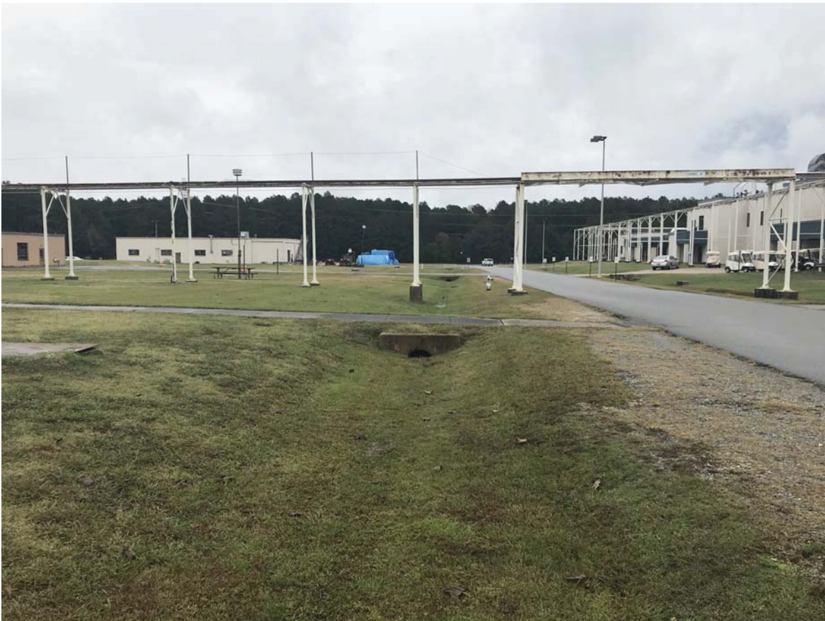
PHOTOGRAPH 3 — VIEW EAST OF LINEAR DRAINAGE DITCH. APPROXIMATELY 1” OF RAIN OVER THE THREE DAYS PRIOR TO THE SITE VISIT.
