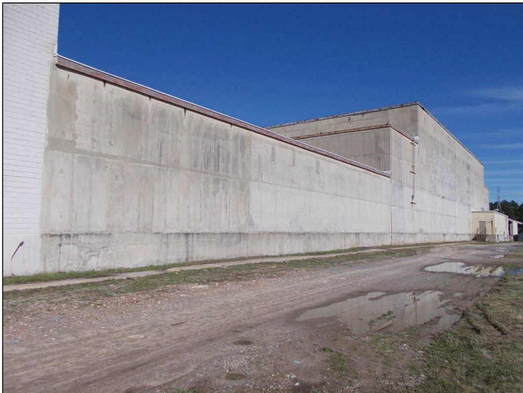
Figure 5-16. Buildings 85C, 85B and 85A south façade, view northeast (DSCN1577).
