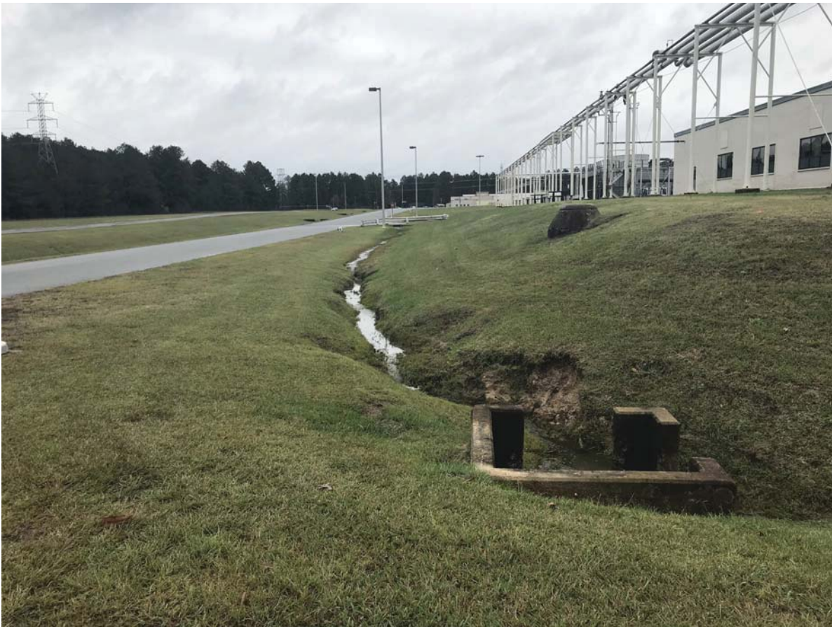
PHOTOGRAPH 7 — VIEW SOUTH WHERE LINEAR DRAINAGE DITCH TRANSITIONS TO EPHEMERAL STREAM A. APPROXIMATELY 1" OF RAIN OVER THE THREE DAYS PRIOR TO THE SITE VISIT.
