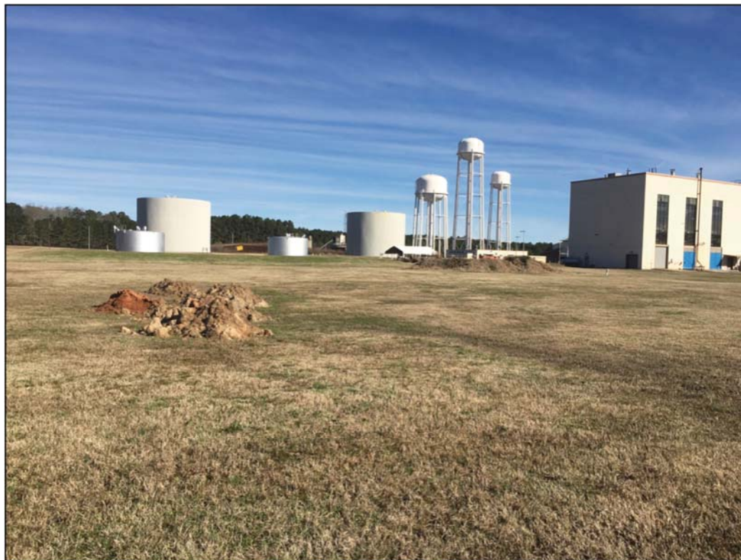
Figure 5-10. Laydown yard north of old railroad grade leading, view northeast (IMG_2271).
