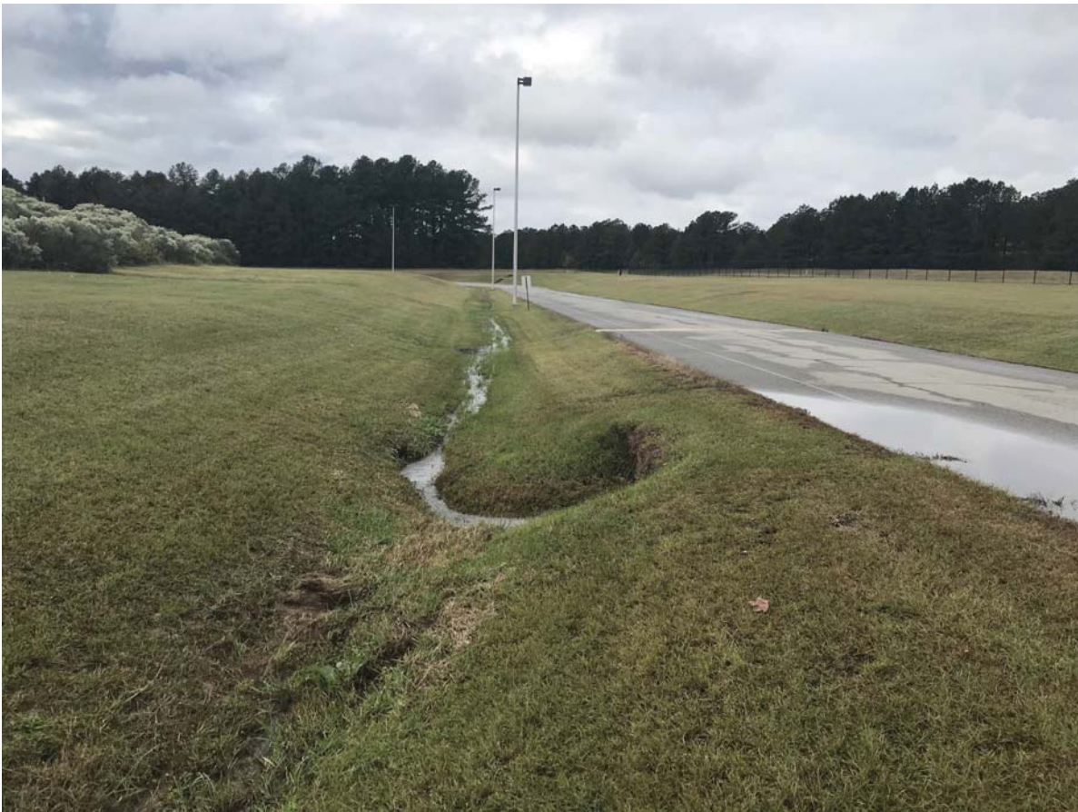
PHOTOGRAPH 5 — VIEW WEST OF LINEAR DRAINAGE DITCH. APPROXIMATELY 1" OF RAIN OVER THE THREE DAYS PRIOR TO THE SITE VISIT.
