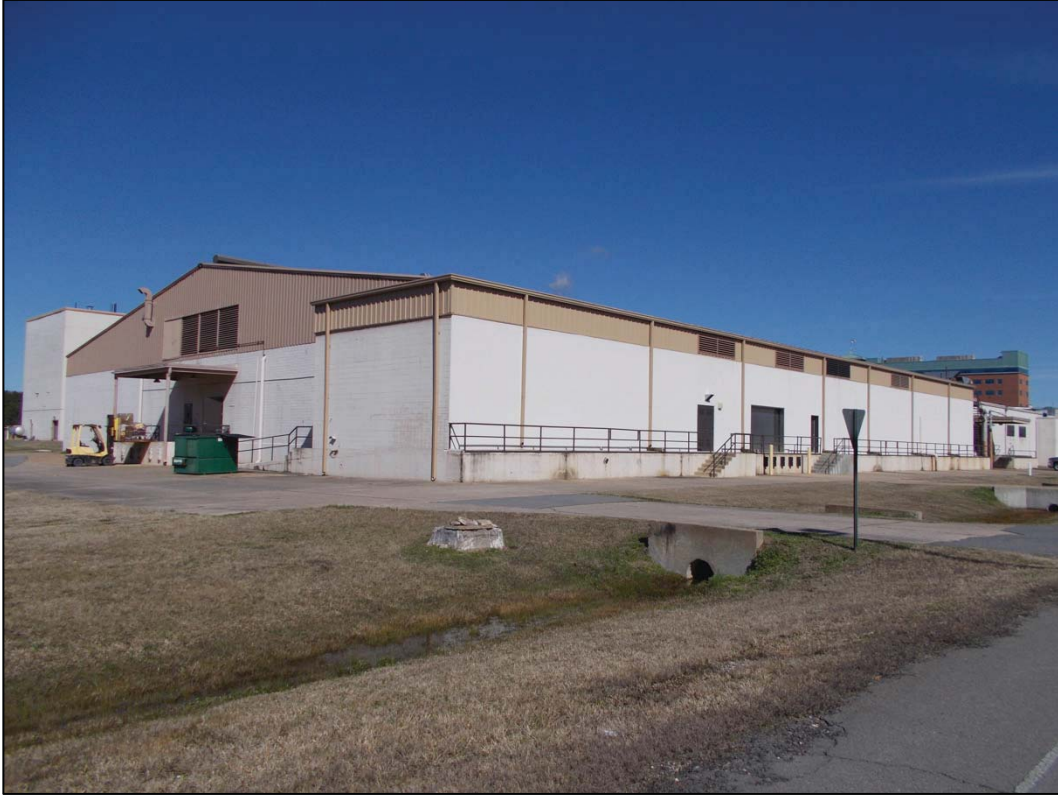
Figure 5-13. Building 5A south and west façades, view northeast (DSCN1573).
