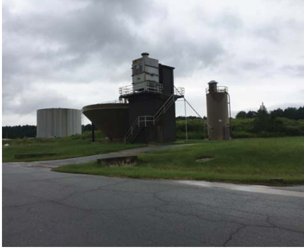
Photo 9: Water clarifier on the northwestern portion of the Campus.
