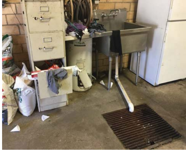
Photo 26: Floor drain in Building 17 (possibly associated with an oil/water separator).
