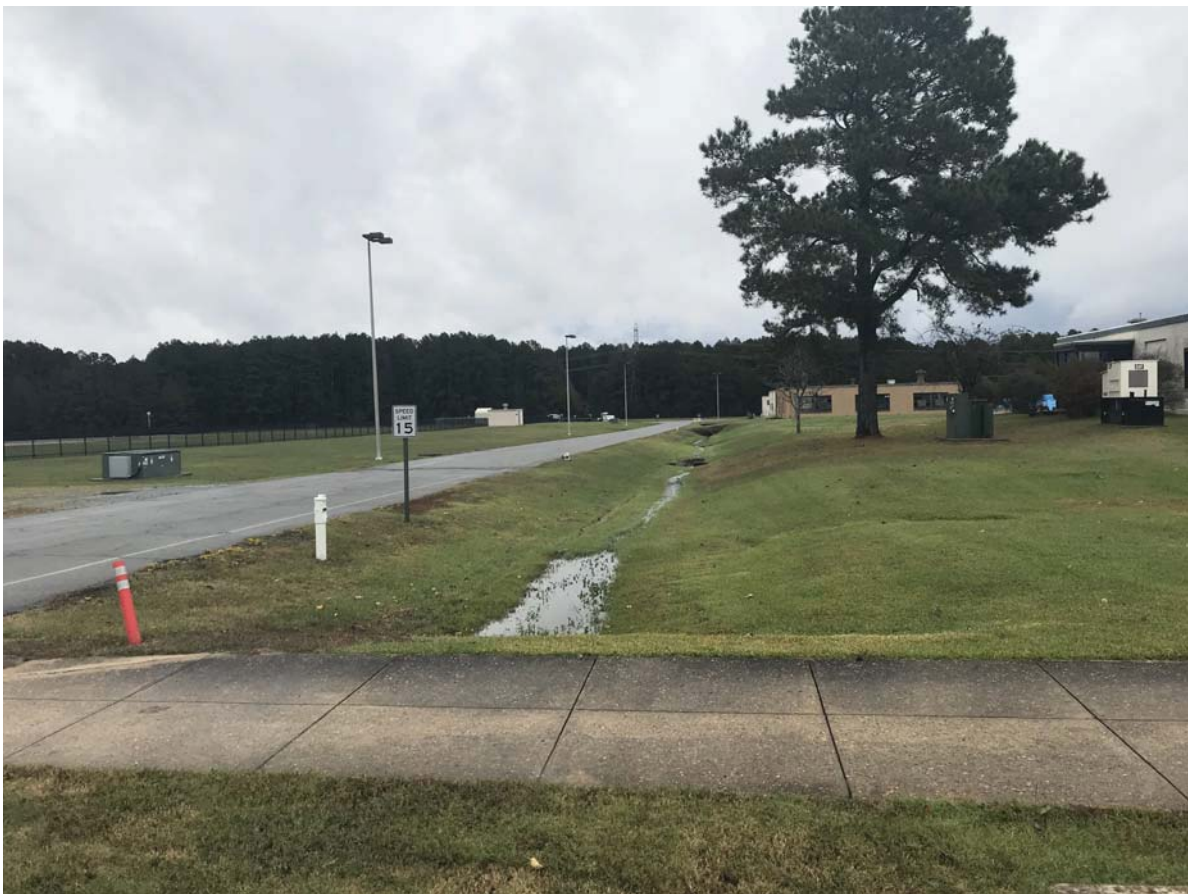
PHOTOGRAPH 1 — VIEW EAST OF LINEAR DRAINAGE DITCH. APPROXIMATELY 1" OF RAIN OVER THE THREE DAYS PRIOR TO THE SITE VISIT.
