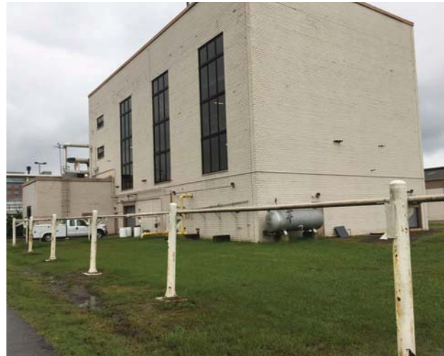
Photo 12: Building 07 (boiler house).
