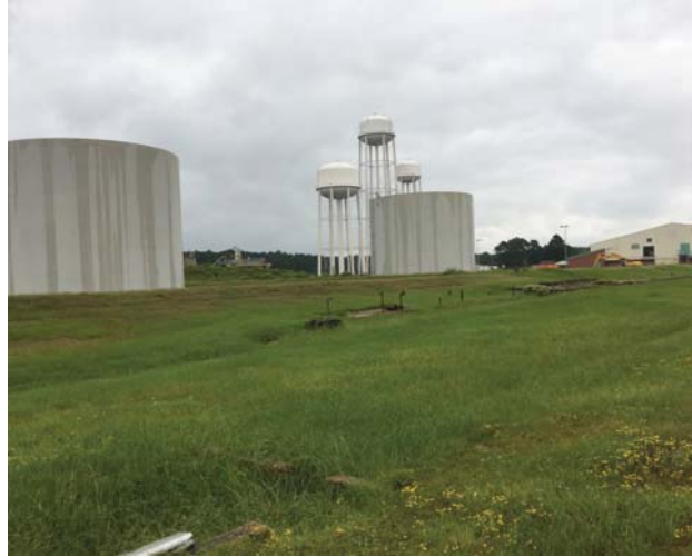
Photo 10: 1,000,000-gallon ASTs (out of service), oil/water separators and water towers on northwestern portion of campus
