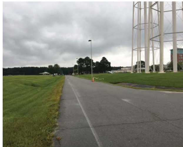
Photo 4: Daniel Road along the northern perimeter of the Campus.
