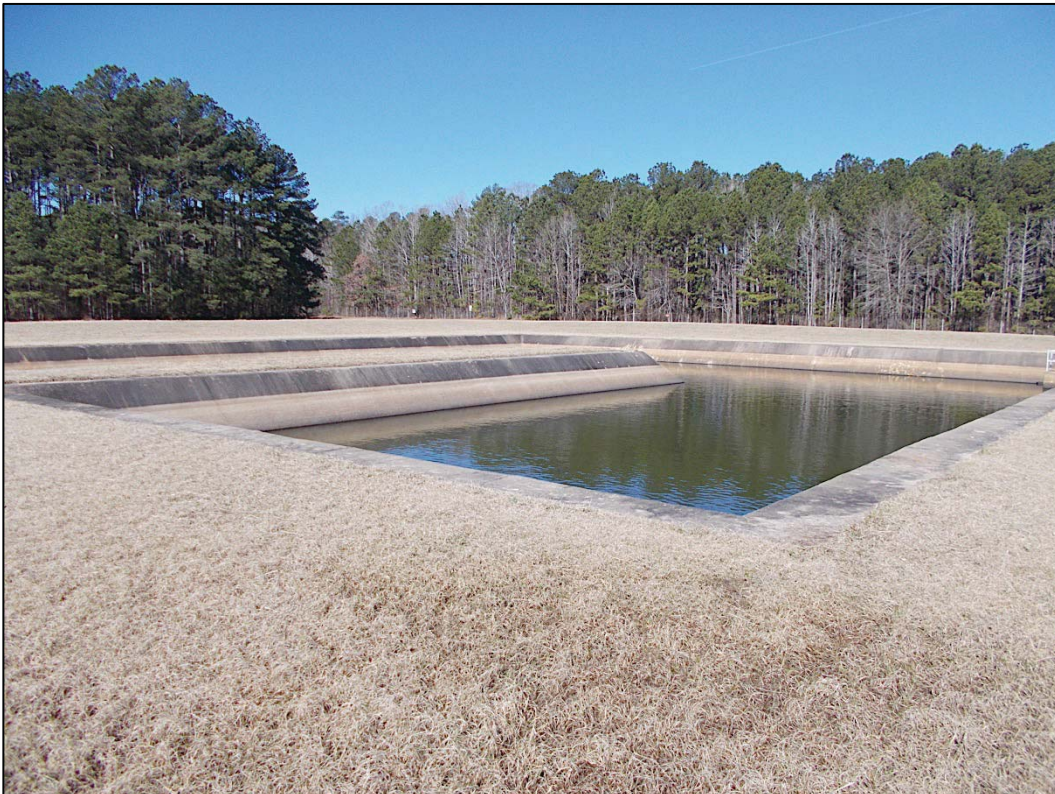
Figure 5-12. Outside perimeter, concrete pond, view northwest (DSCN1623).
