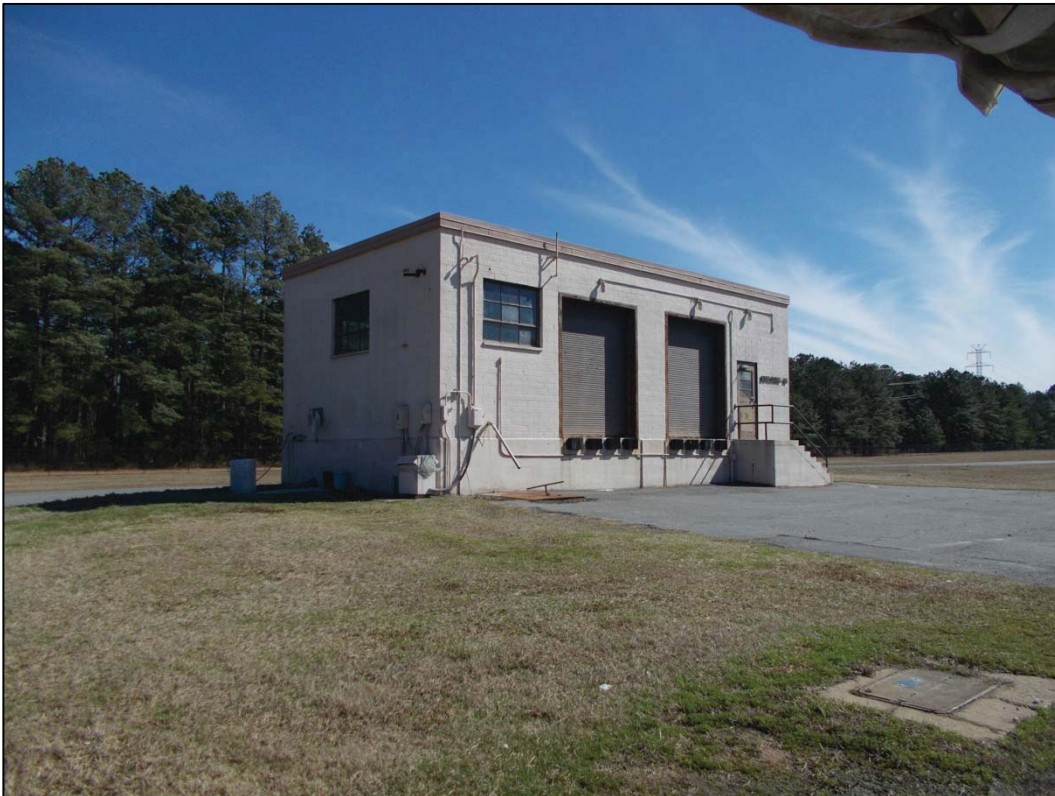
Figure 5-21. Building 16 north and west facades, view southeast (DSCN1560).
