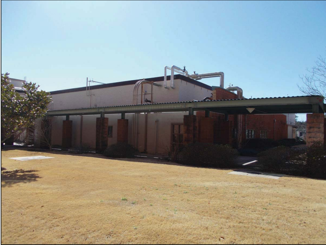
Figure 5-26. Building 51 east façade, view southwest (DSCN1590).
