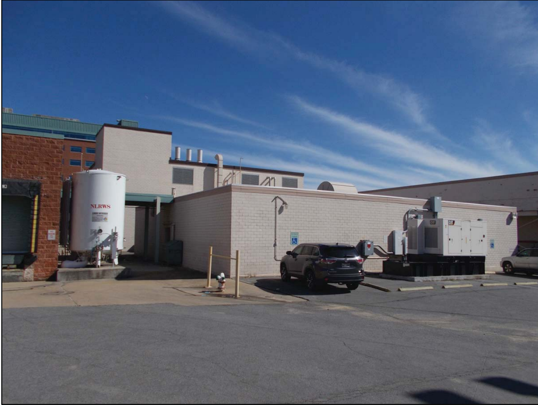
Figure 5-28. Building 60 west façade, view east (DSCN1569).
