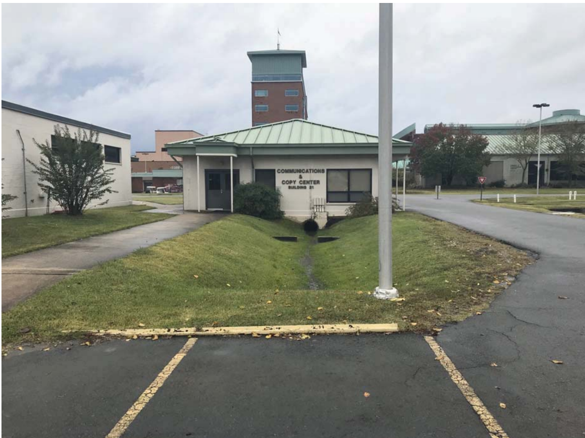
PHOTOGRAPH 2 — VIEW SOUTH OF LINEAR DRAINAGE DITCH PIPED UNDERNEATH EXISTING BUILDING. APPROXIMATELY 1" OF RAIN OVER THE THREE DAYS PRIOR TO THE SITE VISIT.
