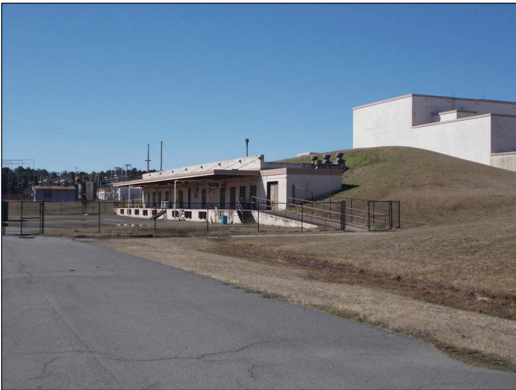
Figure 5-18. Building 37 (Bunker) south façade, view northwest with Buildings 85B-C in the background (DSCN1578).
