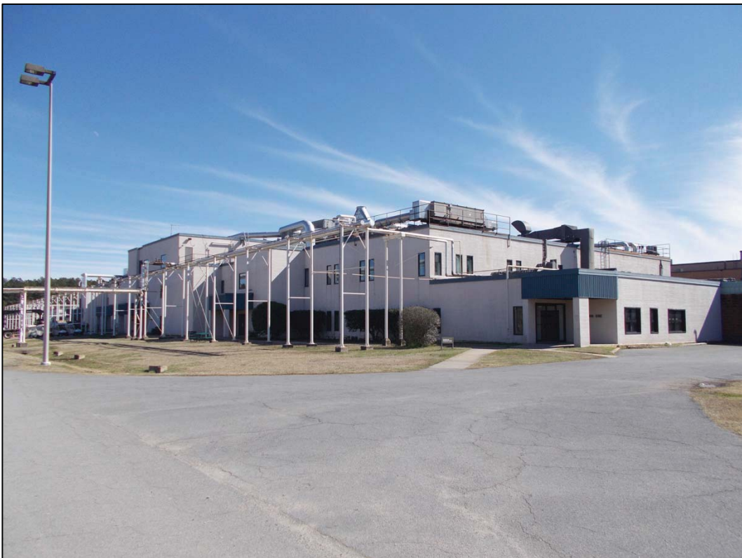
Figure 5-27. Building 53A-E complex (Showers) north façade, view southeast (DSCN1562)
