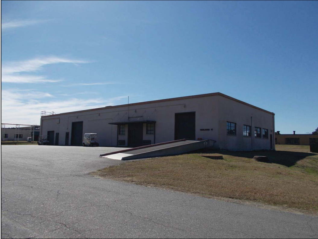
Figure 5-22. Building 17 north and east facades, view southwest (DSCN1559).
