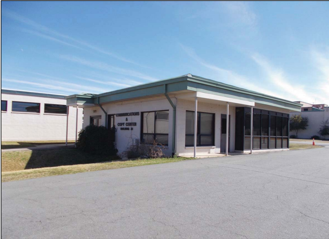
Figure 5-24. Building 31 (Communications and Copy Center) north and west façade, view southeast (DSCN1555).
