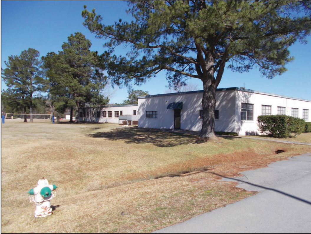
Figure 5-20. Building 13 (Administration) west façade, view northeast (DSCN1556).
