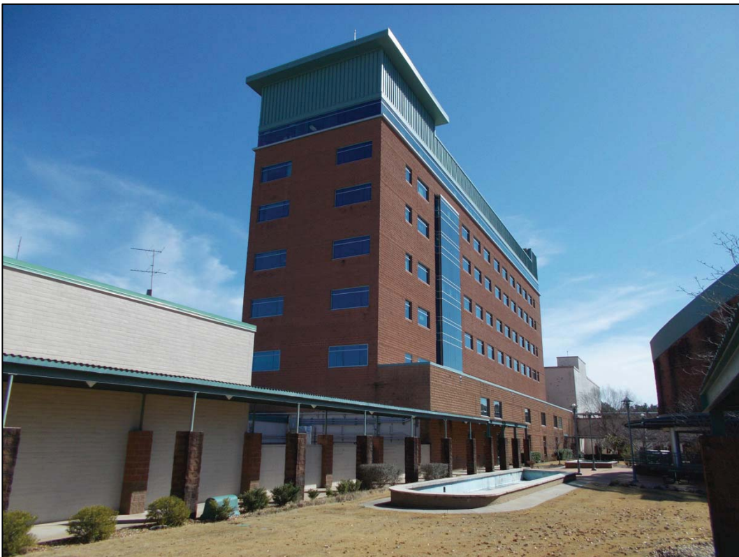
Figure 5-31. Extensively renovated Building 50 west façade, view southeast (DSCN1588).
