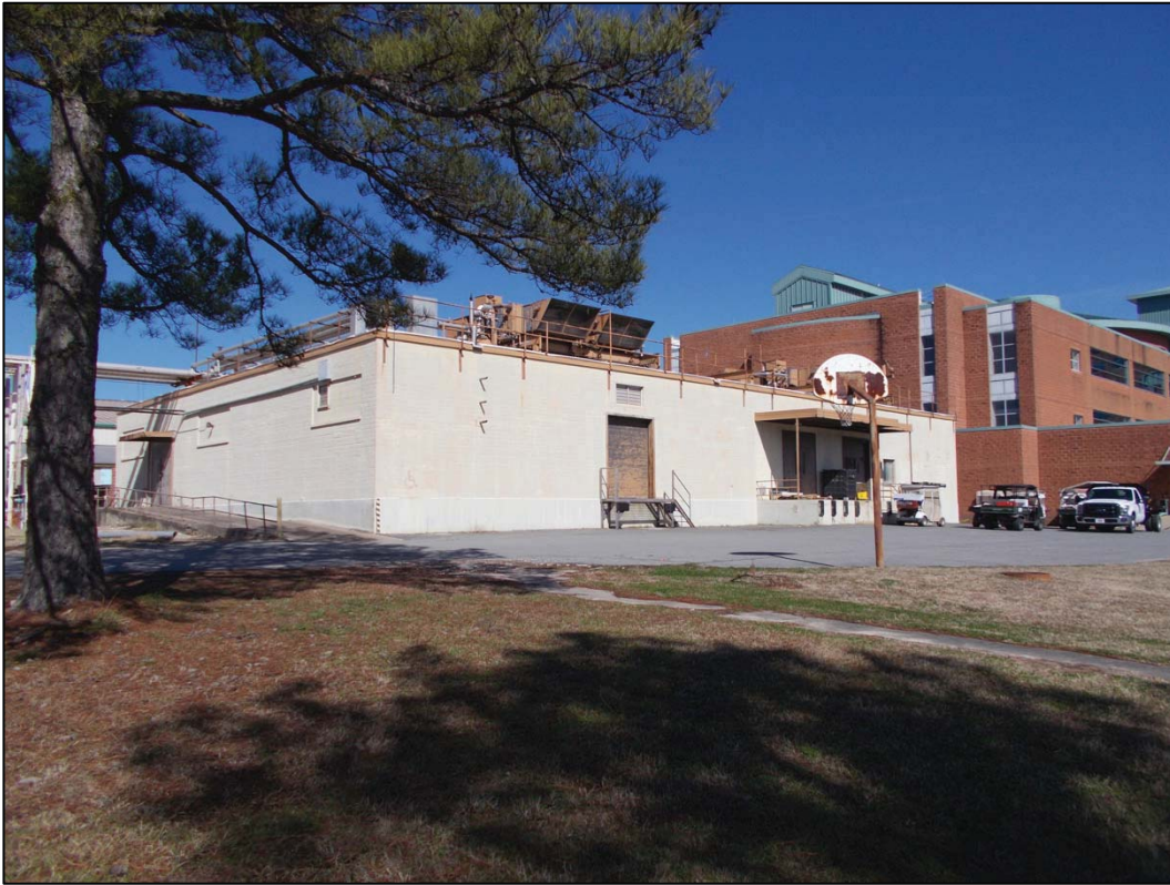
Figure 5-19. Building 6 south and west façades, view northeast (DSCN1568).
