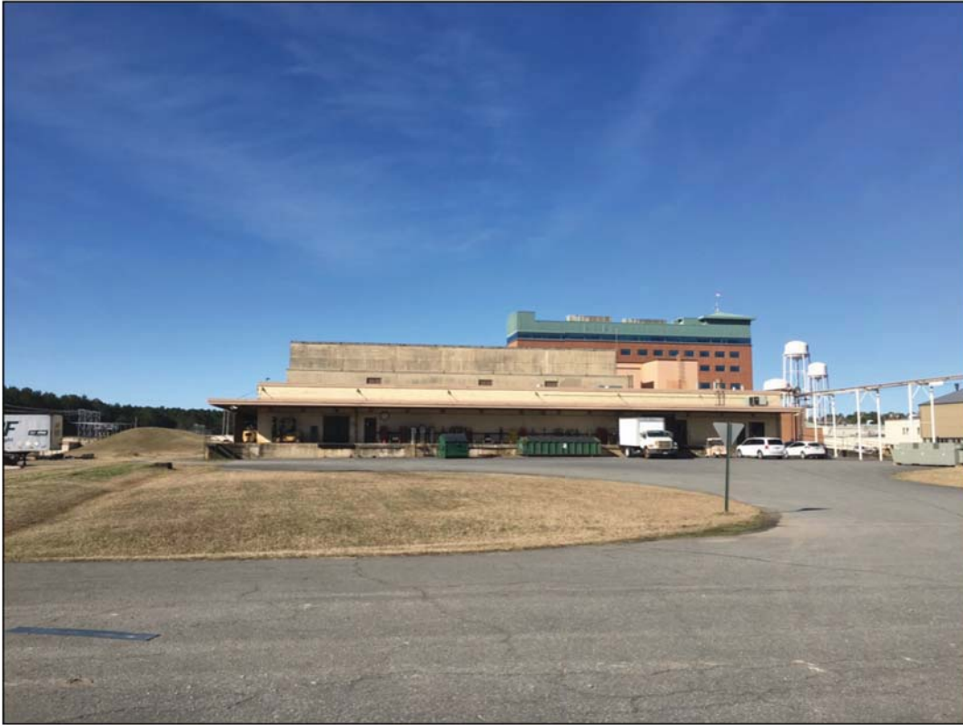
Figure 5-15. Building 85A east façade, view west; renovated Building 50 in distance (IMG_2277).
