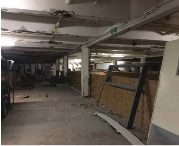
Photo 37: Interior of Building 52.
