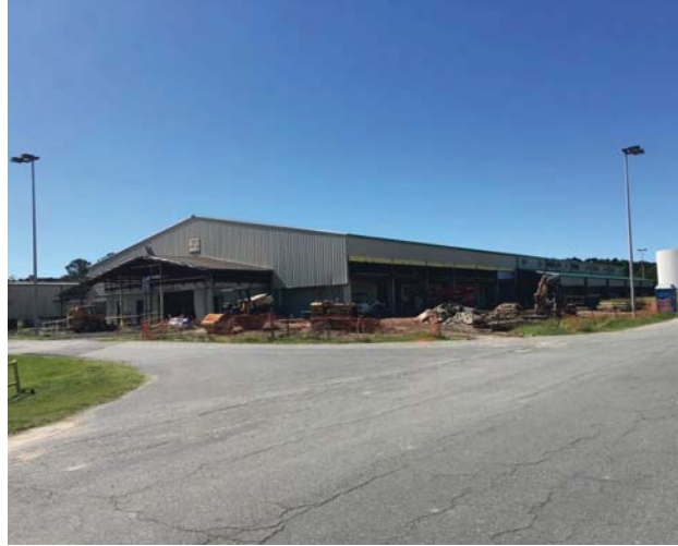
Photo 14: Building 14 (under construction).
