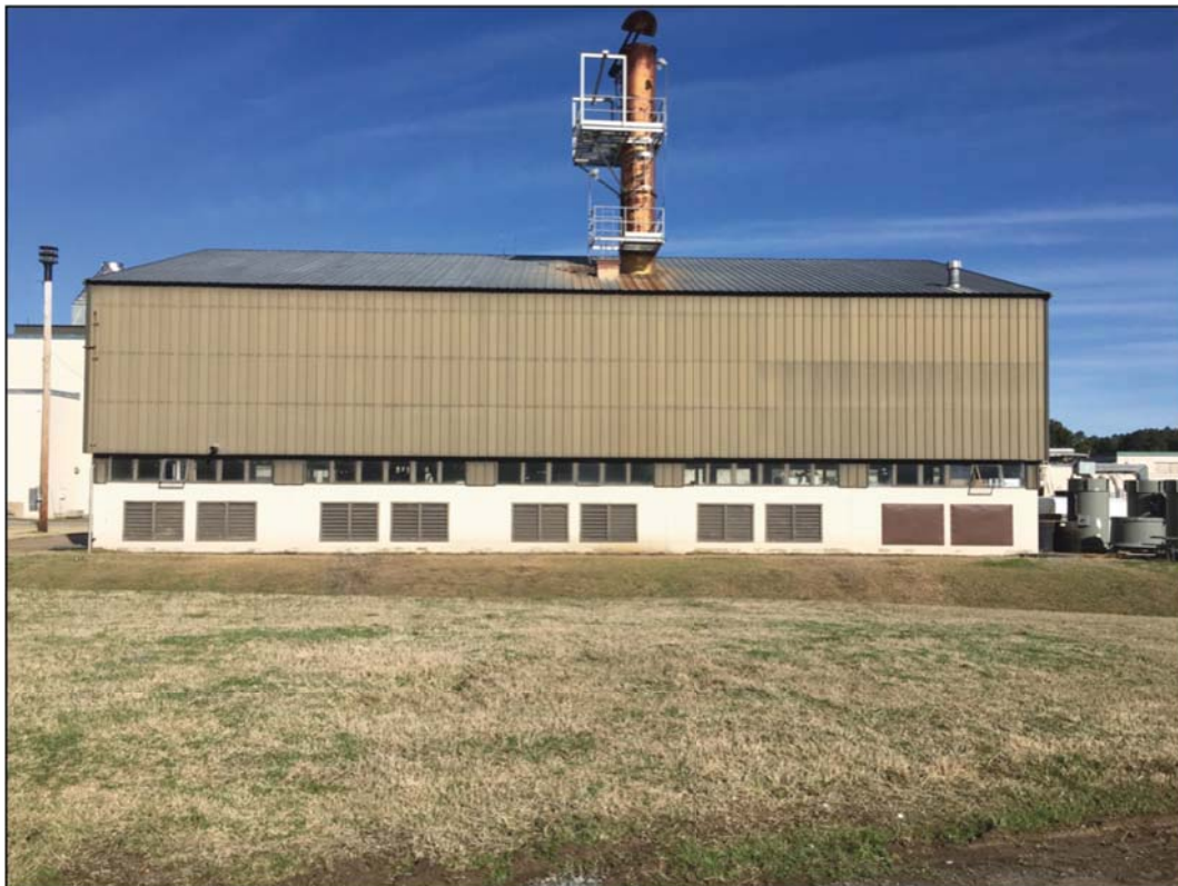
Figure 5-25. Building 46 south façade, view north (IMG_2278).
