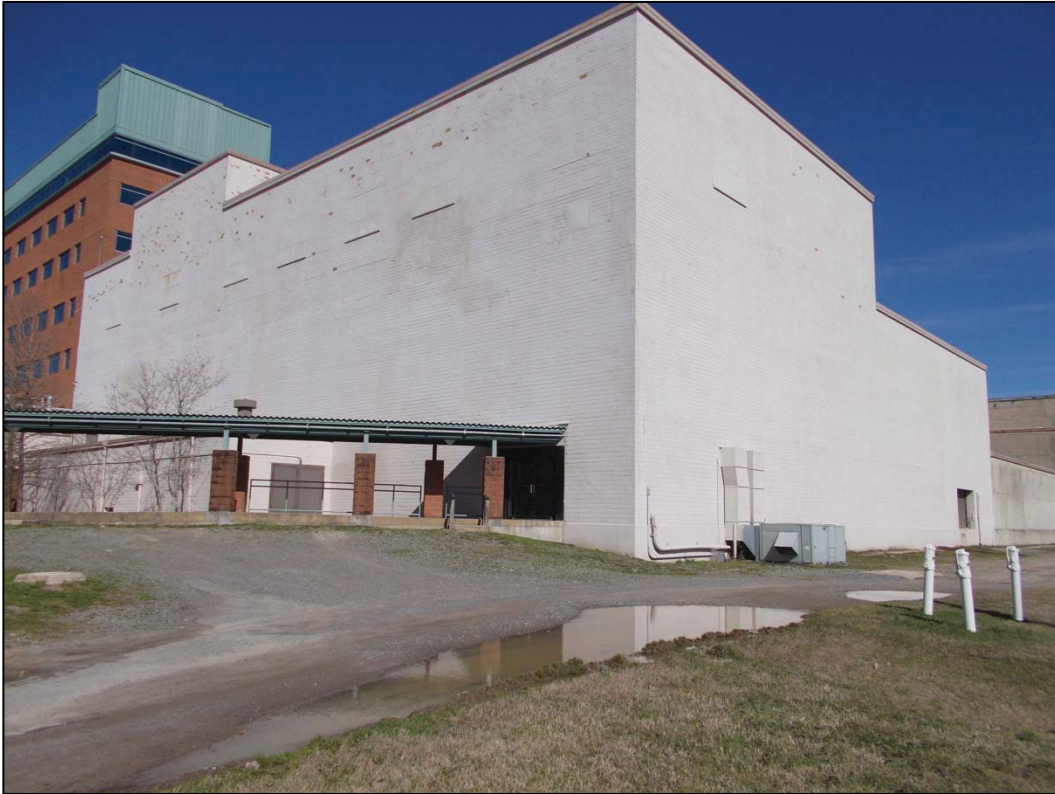
Figure 5-17. Building 52 south and west façades, view northeast (DSCN1576).
