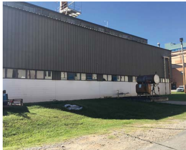
Photo 32: Building 46 and two ASTs.
