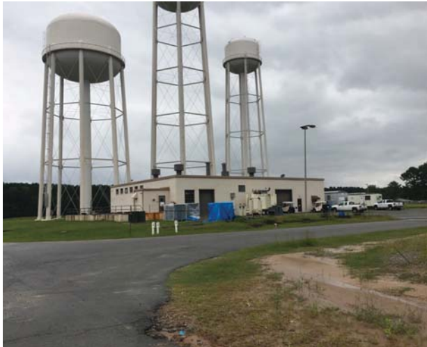
Photo 7: Building 11 (water treatment building).
