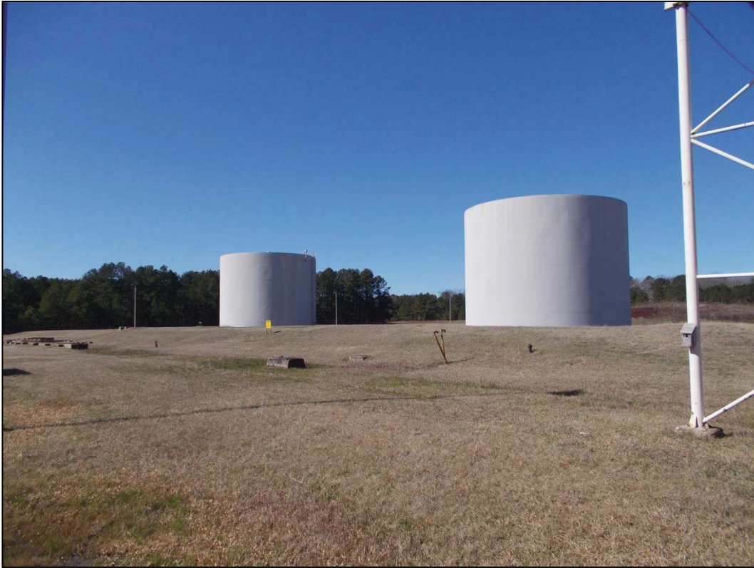
Figure 5-30. Storage tanks, view northwest (DSCN1571).
