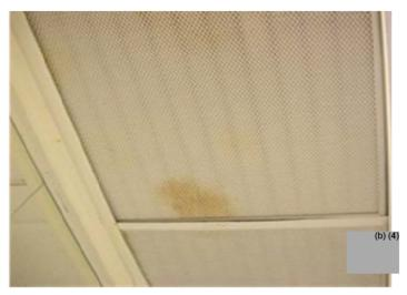
The HEPA filter located immediately above the ISO 5 workbench was observed to have been stained on the filter surface
