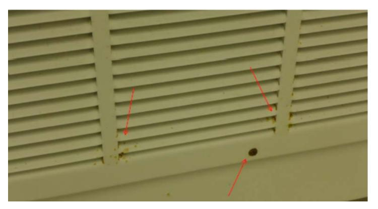
Soiled material was observed on the metal grate covering the pre-filter of the ISO 5 LFH.
