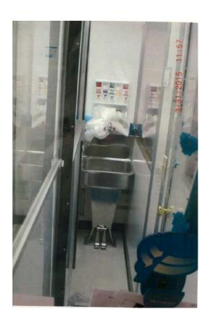
The firm's ISO 7 anteroom design is not adequate. The ISO 7 anteroom is 20 inches in width. Personnel could not gown without touching the walls and the sliding door of the ISO 6 clean room.
