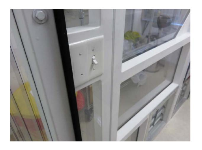
The clean room's positive pressure air handling system was observed to be turned off.
